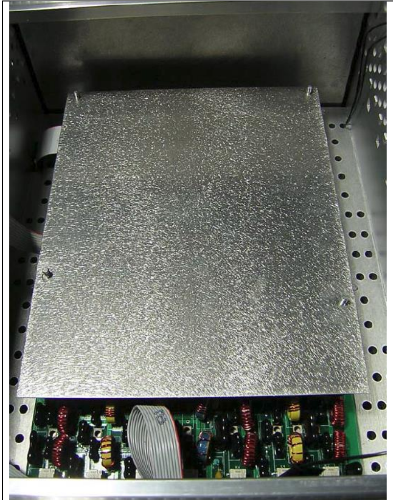
Figure 6 - Placement of RF shield on top of 3/4" spacers
